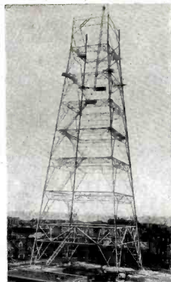
WOR-TV's Tower Construction
